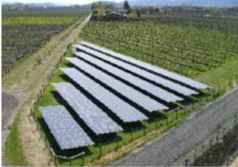
*Honig's solar power system—or their "electricity farm" as they like to call it—is one of the largest in Napa County. The 146 kW system consists of 819 modules, generating 100 percent of their power.*
